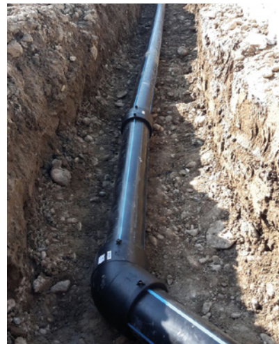
Laying of the hose into the digging.
