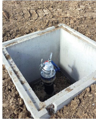
Cement pit with galvanized steel cover for the protection of water intakes.
