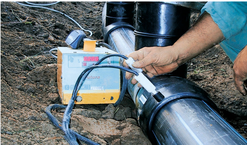
Welding example of electric welded PE hoses.
